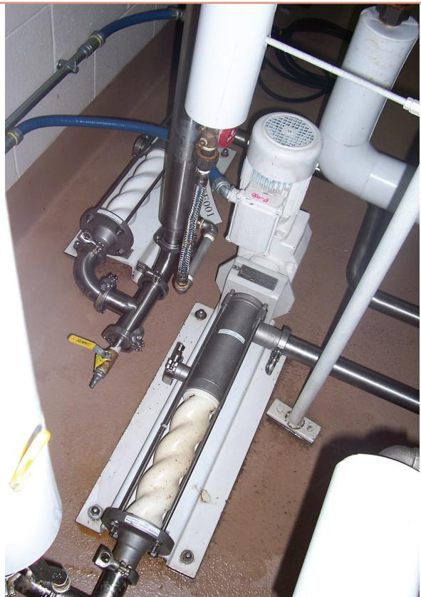
NECCO had been relying on traditional positive displacement pumps to transfer their Sky Bar® fillings from storage to fill line. But, even as they began planning their expansion, design engineers encouraged management to consider progressive cavity (PC) pumps for their new facility.
